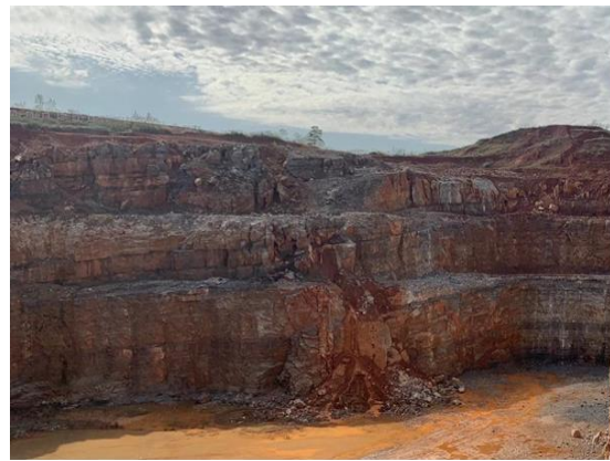
Steep Slopes of Wanxin Quarry (Partial View 1)
