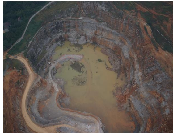
Rockfall Hazard Site in Block E of the Steep Slopes of the Wanshun Mining Pit
