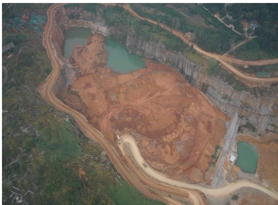
Steep Slopes of the Wanxin Mining Pit
