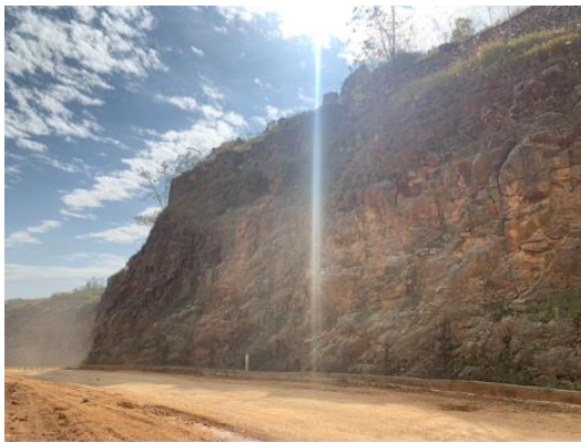
Steep Slopes of Wanxin Quarry (Partial View 2)
